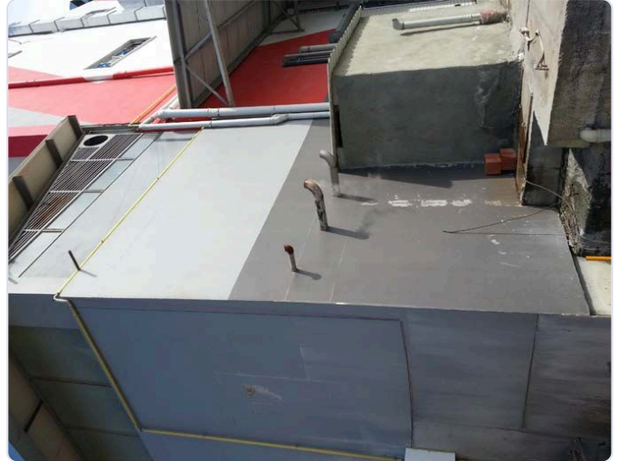
The same vents with the closed cycle and thermocompressors: no plume.
